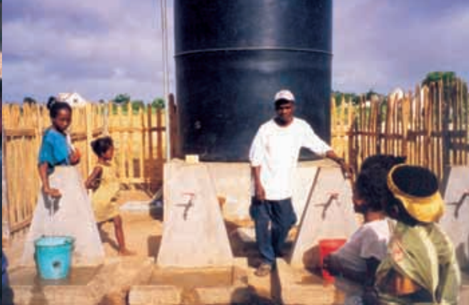
Des bornes-fontaines, installées devant les réservoirs, permettent la distribution de l'eau potable. / Drinking fountains, installed in front of the water tanks enable drinkable water supply.
